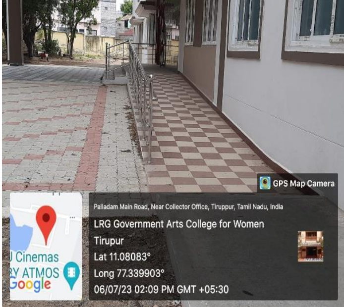
Ramp at Main Building
