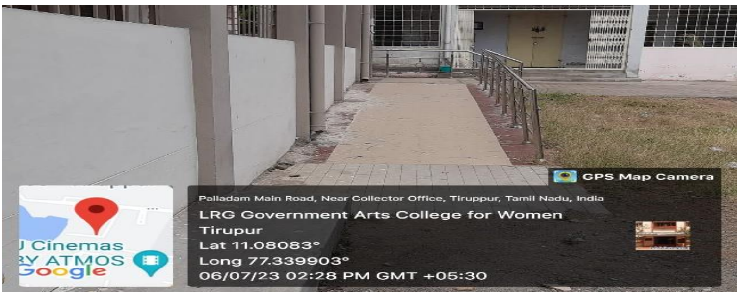
Ramp at R Building
